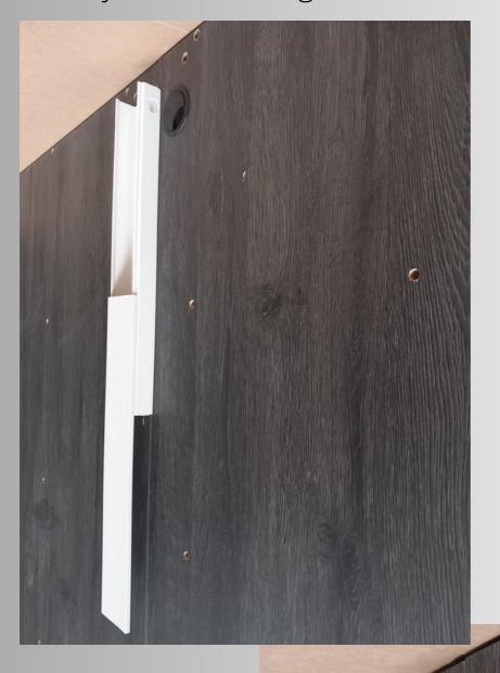
• Fix the cable tray to the revolving panels
